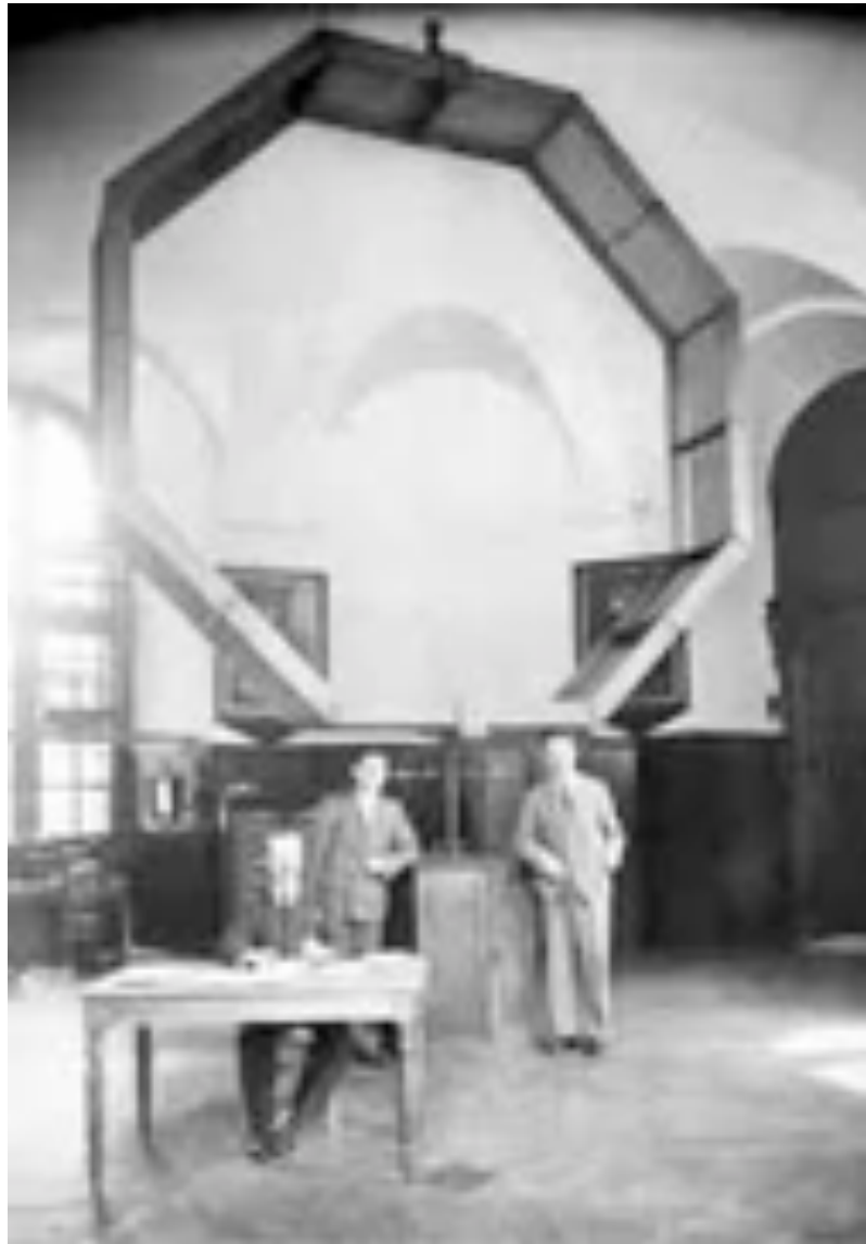
Antenna receiving time signals at BIH
